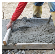
Driveway / Sidewalk Contractors
